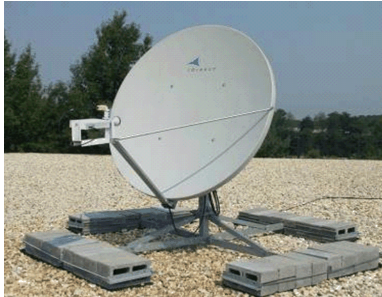
Figure 7 Typical Antenna with BUC and LNB
