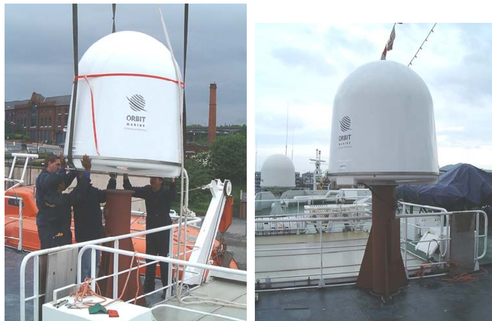
Figure 6-15: Installation on a Vessel
