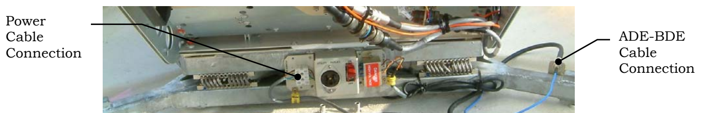
Figure 6-18: ADE Cables Connections
