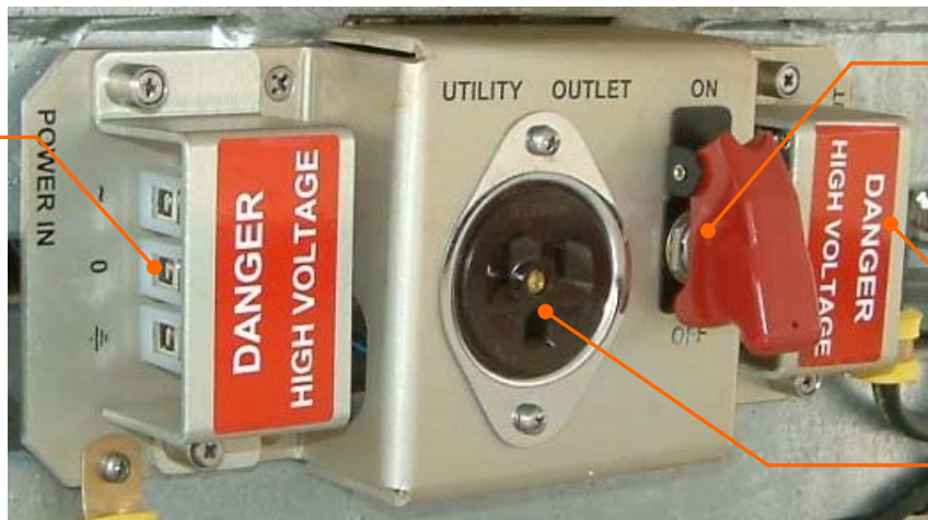
Figure 6-20: ADE Power Connection Box – Original Configuration
