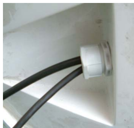
Figure 6-19: ADE Pass-Thru Opening and Gland
